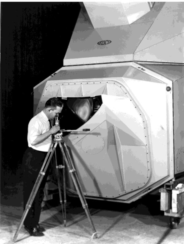
Seen at left is one of the Infinity Display Projectors that fit over the LEM simulator. A separate unit was required for each window of the spacecraft. You can imagine why the astronauts affectionately dubbed the full collection of simulators for the Apollo mission “The Great Train Wreck!”
